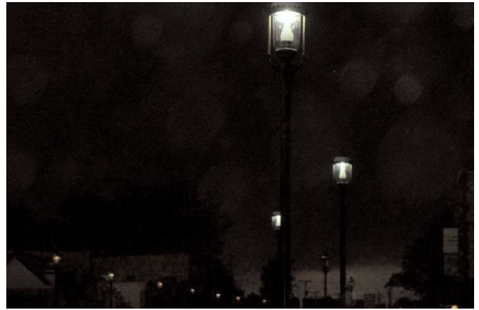
The historic light fixtures have been re-installed on the north side of Lockport Street with an updated light source. The new fixtures provide improved light distribution. The old fixtures can be seen in the background on the south side of Lockport Street.
